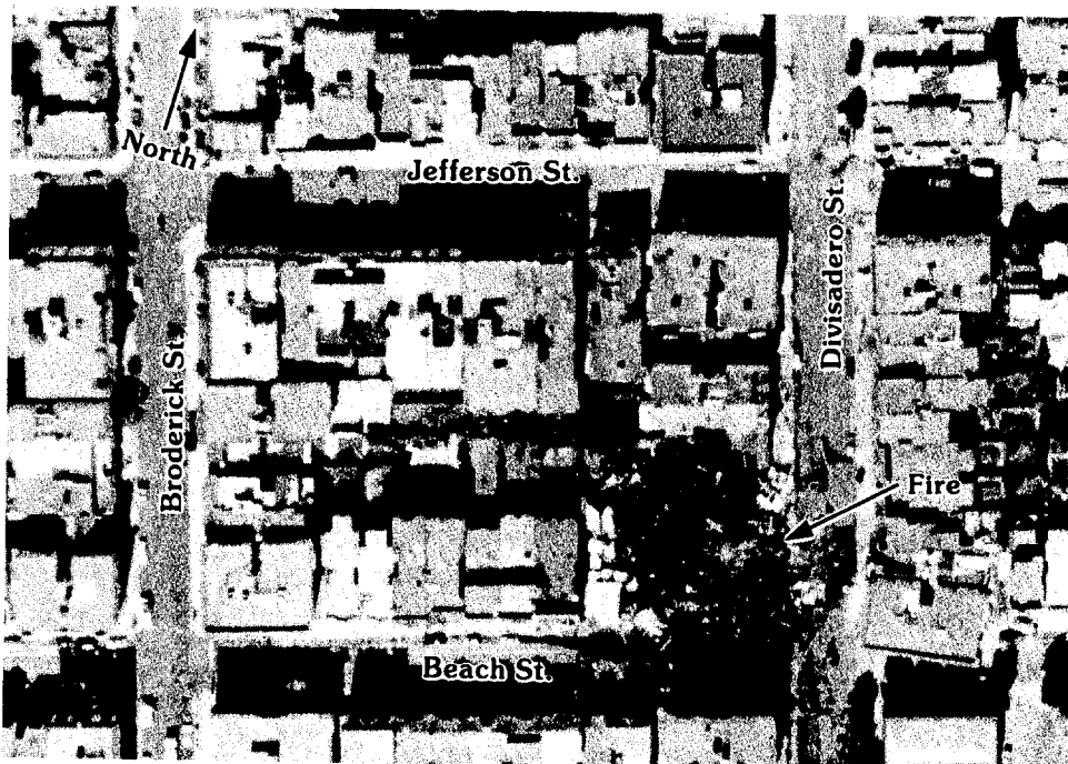
Figure 16.—Northwestern part of Marina District, showing area near Beach and Divisadero Streets. Fire destroyed corner building, another immediately to west, and two more immediately to north.
