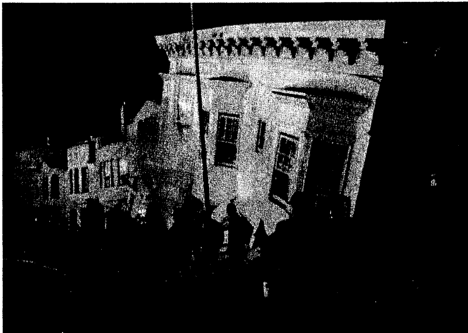
Figure 11.—Collapsed building at 2090 Beach Street, after fire was much advanced. Note firefighter directing water onto exposed side of building. Photograph by S.P. Harris, taken at about 7:00 p.m. P.d.t. October 17, 1989.
